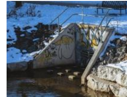
Storm and sewer
