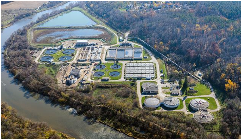
Region of Waterloo Wastewater Treatment
