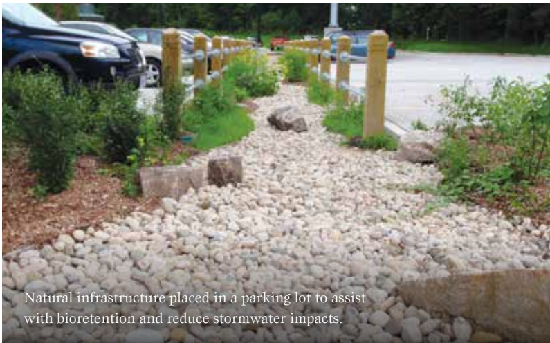
An example of natural infrastructure installed to reduce urban flooding on commercial land. Right: This map highlights the pervious surface areas within the Pearson Eco-Business Zone.
